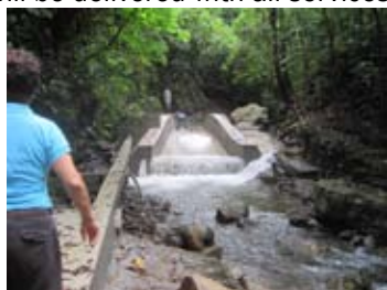
Sylvaine inspecting the progress on the water collection system
