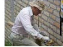
Tim bending rebar at a Habitat home in Honduras.
