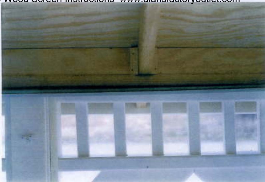
Photo Of Screen Boards & Blocks At Jack Rafter.
