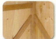
Oak Post & Beam-Style Framing
