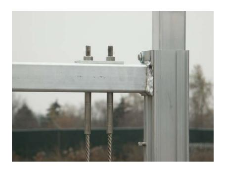
18: Attach the 5/16 carriage bolt, washer, and nut to the lower cable angles. Repeat this for all (4) angles.
