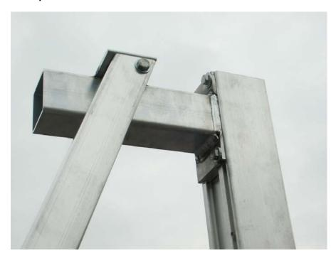
10: Attach V Brace as shown below. Fasten bottom Winch brace first with  $3/8 \times 4.5$ " screw, washers on both sides, and brass hex nut. Keep this screw loose for now. Attach Brace to Winch using  $3/8 \times 1.5$ " screw, washer and brass hex nut. Brace is positioned between Winch plates, fastened to the outside plate.
