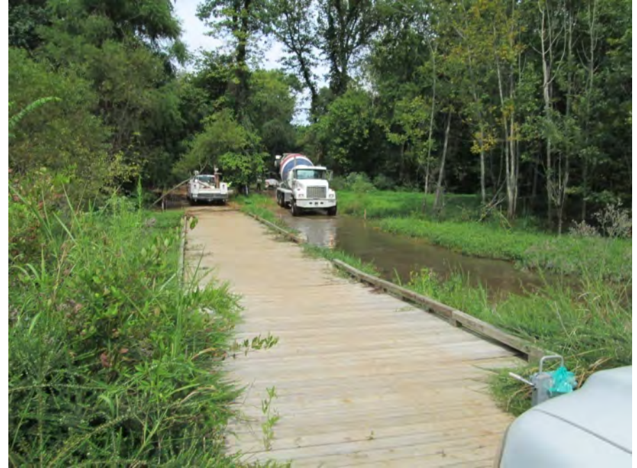
Temporary Access Corridor
