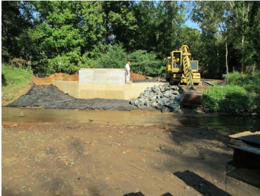
Rip rap placement
