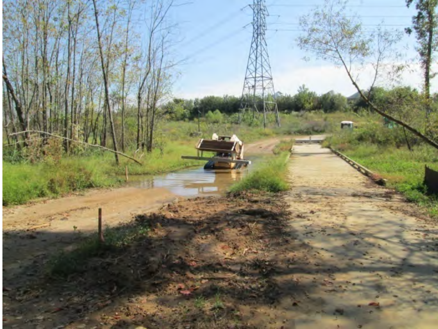
Time to construct ramps
