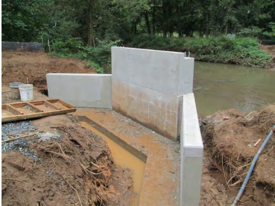
Move forms to opposite bank
