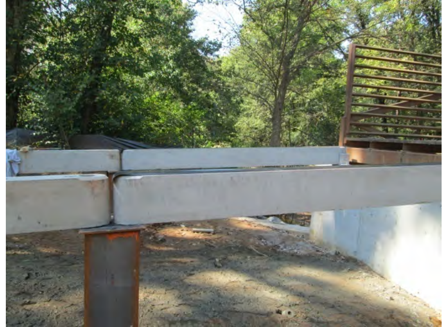
Note welded pilings caps
