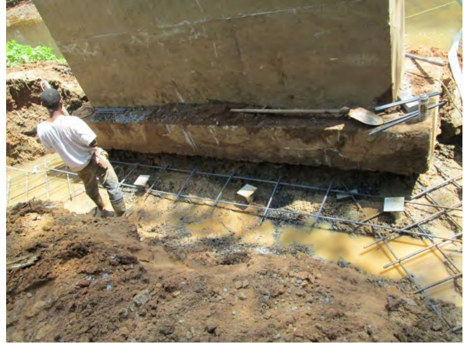
Note helical pier caps
