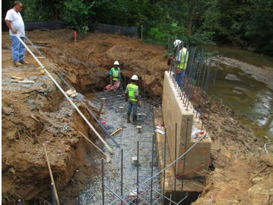
Abutment construction
