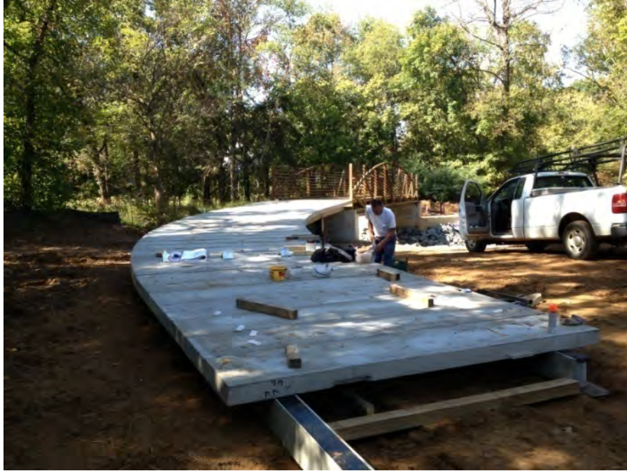
Boardwalk almost to grade
