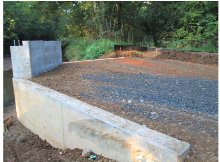
Before and after backfill
