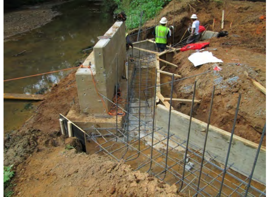
Steel wall reinforcing
