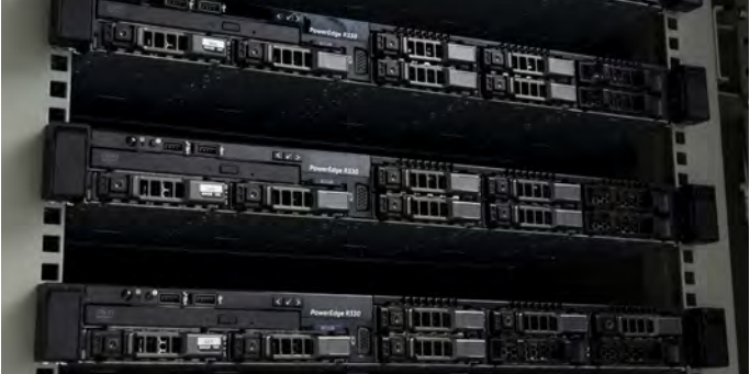
High-capacity and high-speed data server
