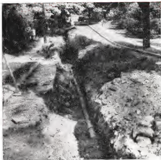
Instolling mechanical joint cast iron pipe for gas distribution main.
