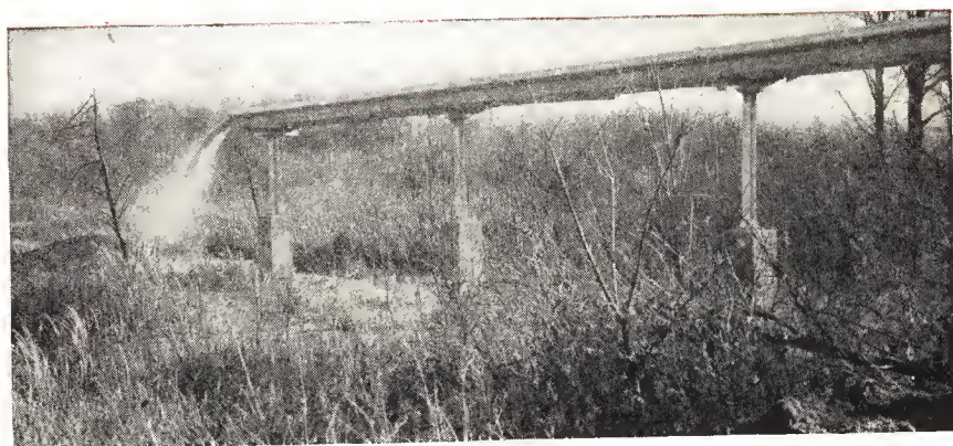
Steam Generating Plants Cast iron pipe carries over 40 tons of ash daily in ash removal system.
