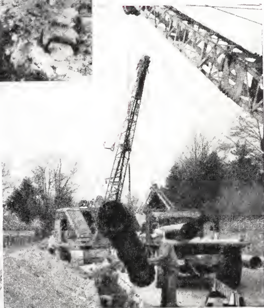
Laying mechanical joint cast iron pipe for a water feeder main.
