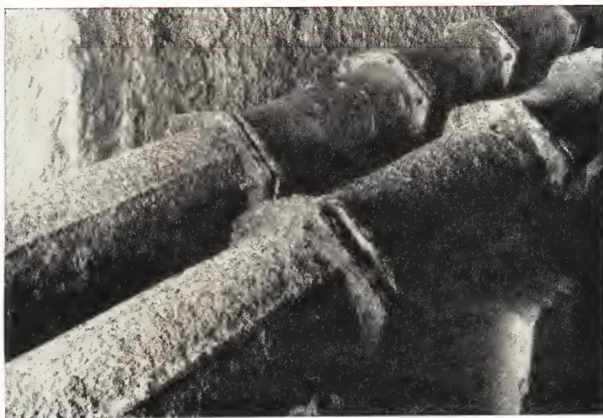
This cast iron water main installed at Versailles, France, in 1664 is still in service
