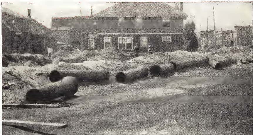
Escanaba, Mich. This 16-inch cast iron pipe, after nearly half a century of service in the water supply system of Iron Mountain, Michigan, was taken up and relaid in Escanaba, about fifty miles away.
