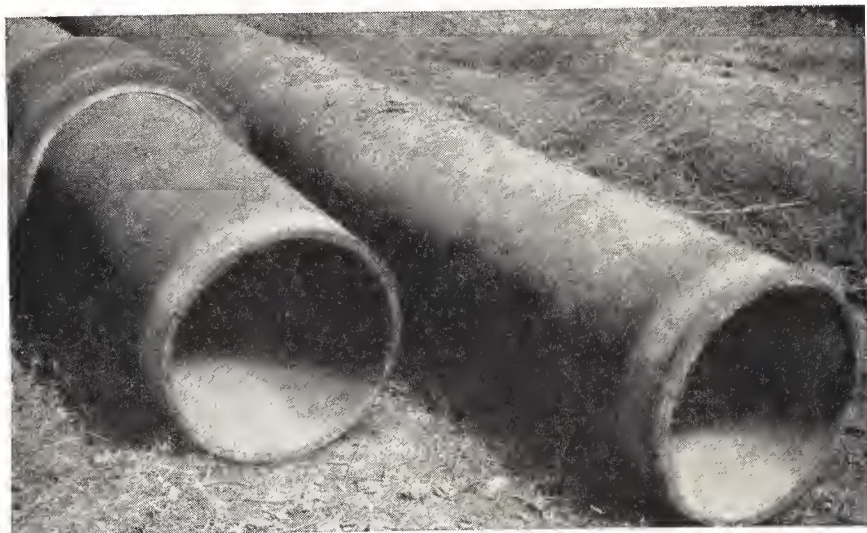
Springfield, Missouri. In connection with changes at a pumping station, part of a 50-year-old 18-inch cast iron water main was recently taken up and relaid in another part of the city. Note cast marks and date clearly discernible on pipe in right center.
