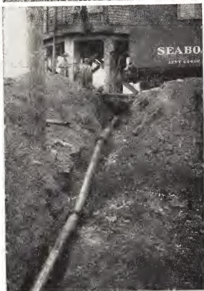
Steam Generating Plants Cast iron pipe carries over 40 tons of ash daily in ash removal system.
