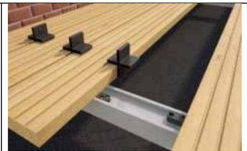
**Step Six:** Choose any of the four spacing options available on the Deck Spacer, Flip the board over and slide it into place. The unfastened end will be held in place by the prior row of decking. Fasten the other end of the Deck Glider to the joist.
