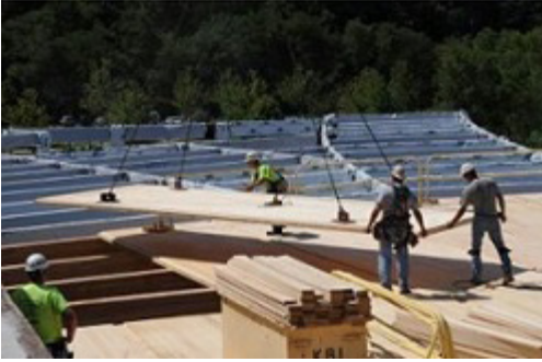
Left: Cross-Laminated Timber roof panel being installed in Madison, Wisconsin. (Photo courtesy of David Kretschmann, Forest Products Laboratory) and Right: Panelized shear wall system. (Photo courtesy of AISC)
