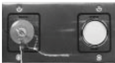
10-1643 Manual Release/System Abort
