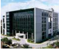
Taoyuan Technology Center (Green Building)
