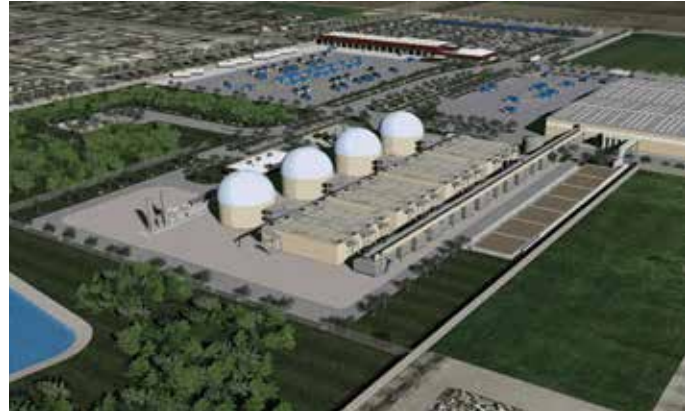
Biogas plant in Perris, USA.
