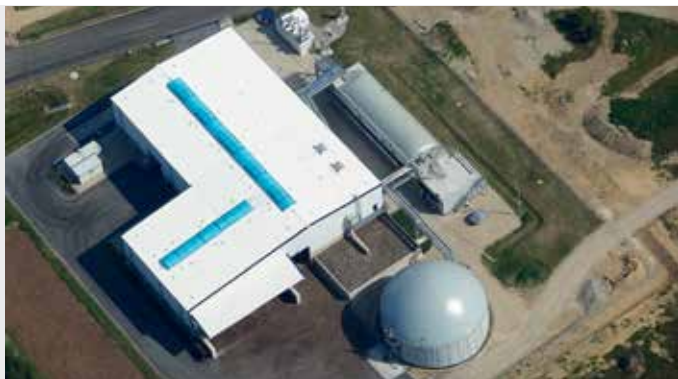
Biogas plant in Schwerin, Germany.
