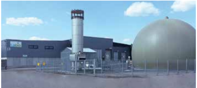
Labio Oy, Finland – our largest biowaste digestion plant in Europe.
