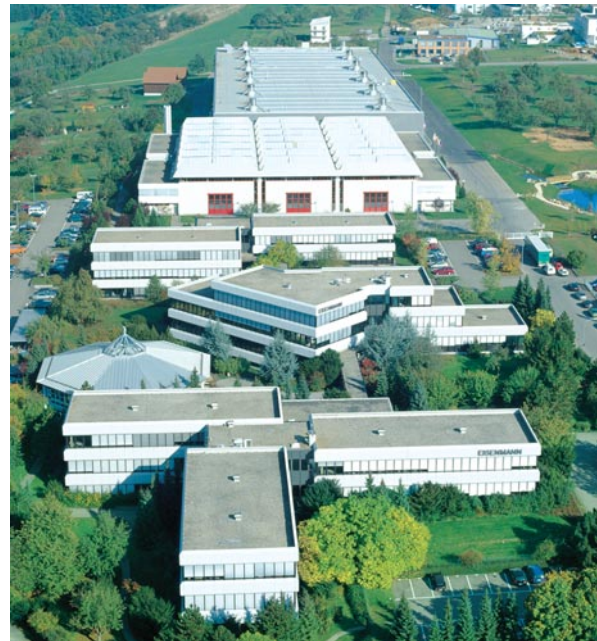
EISENMANN Technology Center in Holzgerlingen
