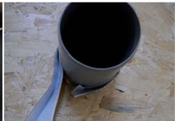
Do not overlap the adhesive tape yet!
