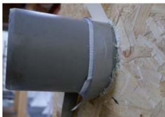
Remove the second sheet of silicone paper
