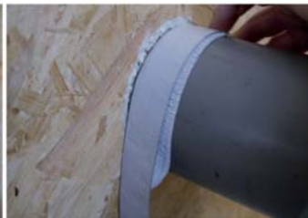
Attach the adhesive tape to the opening
