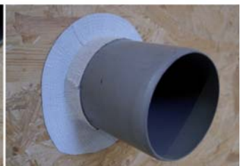
Completely sealed opening
