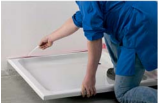
3. Remove upper protection foil.
