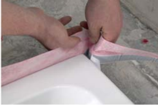
2. Fix the band with noise protection on the rear side of the the tub.
