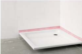
4. Fix on the wall a little over the tub and press to fasten.
