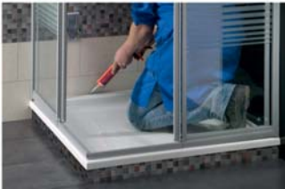
6. Apply silicone joint.
