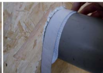
Attach the adhesive tape to the opening
