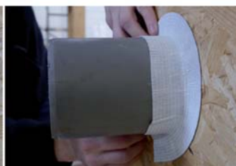
Apply the second side of the adhesive tape to the substrate
