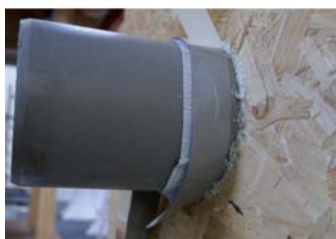
Remove the second sheet of silicone paper
