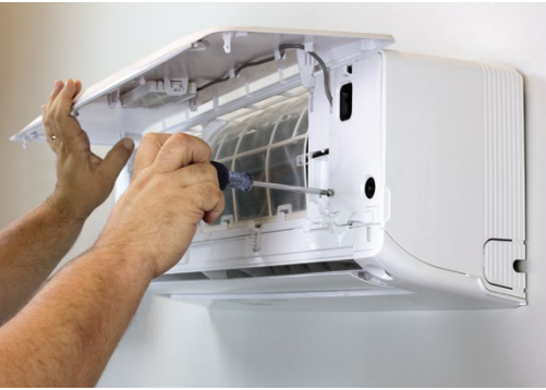
Back out electrical panel screws
