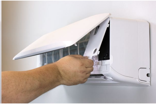
Remove electrical access panels [2]
