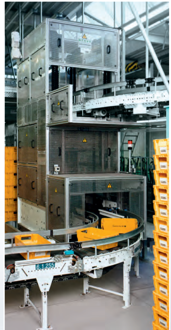
C-conveyor in mail distribution centre
