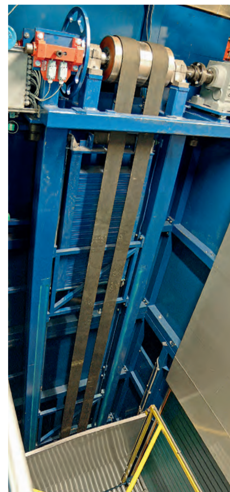
Drive station of heavy-duty reciprocating lift with geared motor, coupling, drive drum and locking mechanism
