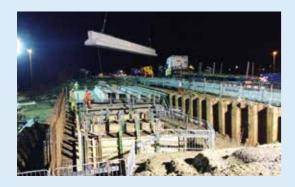
Oxfordshire County Council's work on the Milton interchange is nearly complete. Since January the final concrete beams for the new bridge have been installed, the walls underneath the bridge are being completed with brick cladding and resurfacing of the road above the bridge is underway. You will have also noticed new traffic signals and the continuing construction of the new road which will join the A4130 and A34 northbound carriageway.
