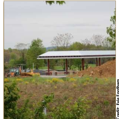
Future Shell station near PHC
