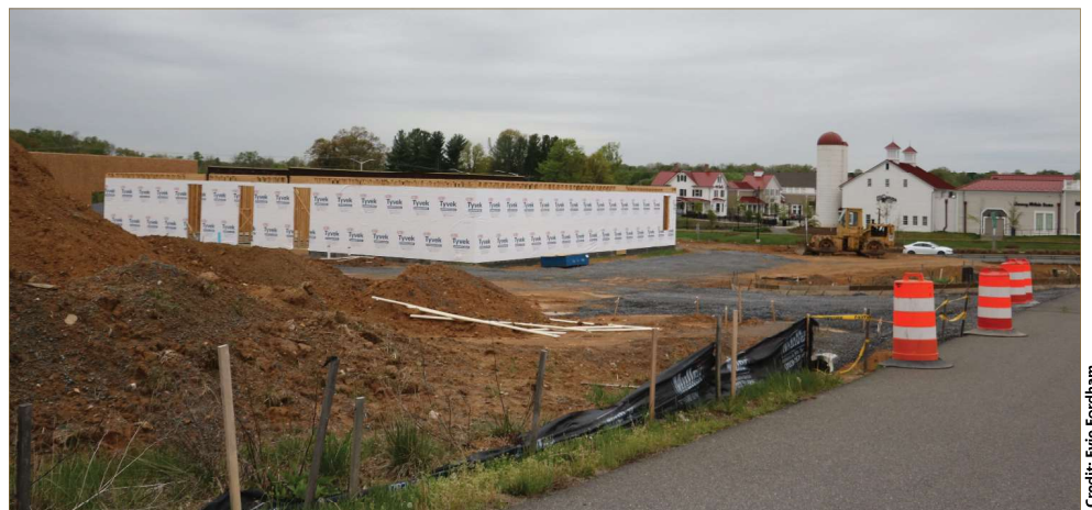
View from BHC parking lot of Catoctin Corner buildings under construction
