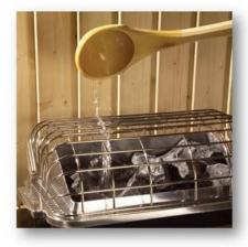
When the high temperature is achieved, the elements cycle on and off to maintain the high temperature. Most traditional sauna users enjoy pouring water over the rocks to create steam to raise sauna humidity levels. The benefits of pouring water over the rocks include: making the room more comfortable, moistening the nasal passages, and allowing the use of aromatherapy by mixing essential oils with the water.
