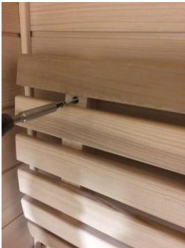
*Note: Be sure to install level to ensure a well-balanced look. Use seam in T&G for reference. Another hint is to place a couple 2x4 cut-offs or blocks of foam packing material that is 8" – 10" high between the upper bench and backrest to establish perfect symmetry between the bench and backrest.*
