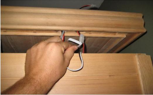
8. Connect the wires in the ceiling panels accessed via flip-up panel as shown above. There are three access doors. Back Right, Right Wall and Front Right.
