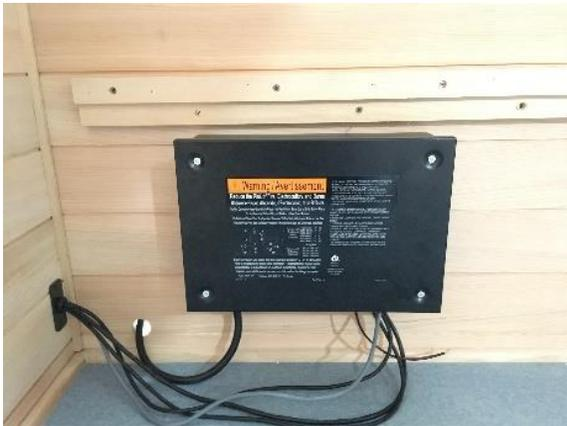
15. Hang heater on front wall. The wall is labeled and predrilled for the top lag screws found in the sauna heater hardware pack. Insert screw so there is about 1/8" gap to the wall bracket. Once the heater is in place, you can tighten the lag screws to secure the heater to wall. For complete security, you may mark and drill for the bottom 2 screws to be installed as well. (Note: you may want to make all electrical connections before final tightening of lag screws.)
