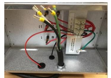
15. Insert the black, white and green wires into the terminal block as shown. Tighten the screws securely (approximately 18 in/lbs.)
