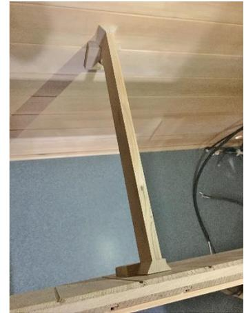
33. Install the bench brace from the back of the Bench Skirt to the back wall.
