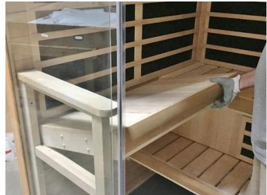
39. Place the return bench squarely onto the pre-installed supports to provide a snug fit. The bench will be supported by the Upper bench support and the Armrest support by the glass wall.
