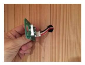
Step 5: Connect the sensor wire coming out of the wall above the heater to the sensor assembly. The sensor will then be fastened to the wall over the hole with a screw.
