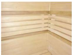
Step 6: Install the backrests above the upper benches according to the predrilled holes, using the 1 1/8" screws provided.
