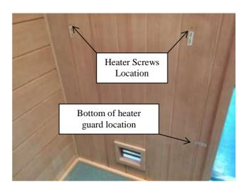
Step 2: Mount the sauna heater according to the Installation and Operation Manual provided with the heater. The wall is labeled and predrilled for the top lag screws from the sauna heater hardware.
