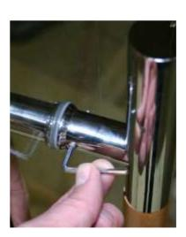
Step 10: Install exterior portion of door handle on the screw section and tighten all four setscrews with Allen wrench.
