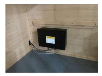
Step 1: Mount the CB-PK-1 contactor box to the right wall with 4 screws provided by locating the lower left corner of the box to wood pencil trim on wall.
