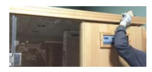
Step 4: Place the ceiling panel on the wall panels.
