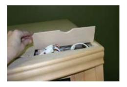
Step 6: Connect the wires in the ceiling panel accessed via flip-up panel as shown above.
