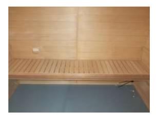
Step 2: Place the lower bench along the wall spanning from left wall to right wall.
