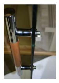
Step 9: Install the handle on the glass. Ensure the plastic gaskets are on both side of the glass while installing the screw into the door handle.
