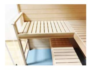
Step 3: Place the return bench squarely onto the pre-installed supports to provide a snug fit. The bench will be supported by the Upper bench wall support and the armrest support by the glass wall.
