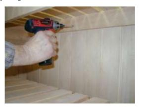
Step 5: Be sure to fasten the upper benches to the walls using the 1 1/8" screws provided. Lower benches are meant to slide on the lower bench supports for cleaning convenience. The bench installation is complete.
