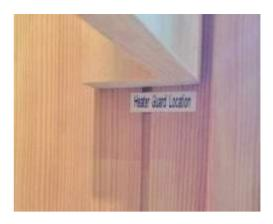
Step 6 Install the wood heater guard around the sauna heater using the 1 1/8" screws provided. The heater guard location is marked on both walls with a label. Place the bottom of the heater guard to cover the label on the walls and secure into location.
