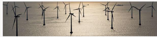
Siemens Wind Power, one of the world's largest wind turbine manufacturers, uses RTI Connex DDS to integrate its entire farm. Wind turbine farms can include as many as 500 turbines with 100-meter blades. Turbine control requires fast local loops and maintenance data collection. Gust control across the array necessitates fast communications with dynamic, selective filtering.
