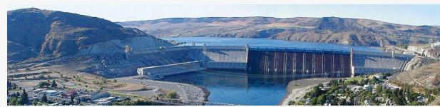
The largest power plant in North America has replaced its SCADA control system with RTI Connex DDS. The aging, monolithic SCADA system was no longer effective at meeting today's important requirements – extreme availability, fault tolerance, performance, security, and ability to implement wide-area communications.
