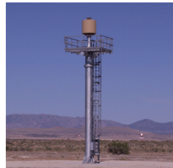
Figure 8: The Ground Based Sense and Avoid (GBSAA) system includes many distributed radars. It will soon allow unmanned vehicles to fly in the U.S. National Airspace System (NAS). Applications of unmanned vehicles will include operator training, repositioning, search and rescue, and disaster relief.
