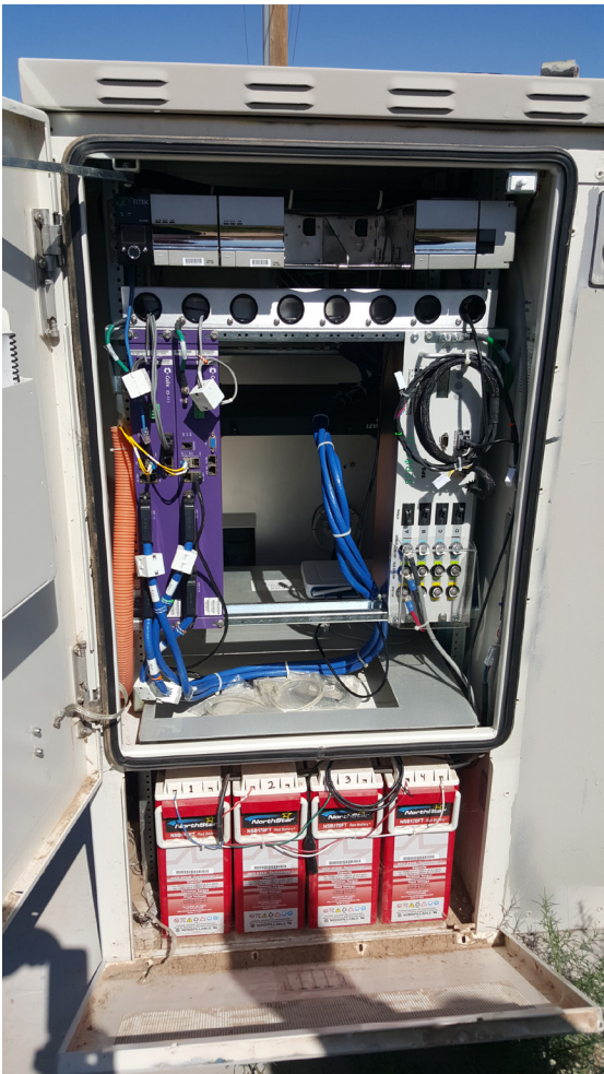
Figure 1: Servato’s Smart Power System (SPS™) (pictured above at right) is capable of measuring battery state of health with unprecedented accuracy in situ . This proprietary function, combined with unmatched data collection and analysis, enables the Servato to extend battery life, predict battery failure, and provide real-time battery information, while also detecting equipment issues like bad rectifiers. The SPS™, along with Servato’s cloud-based software ActiView®, are the basis of Servato’s Active Battery Management.™
