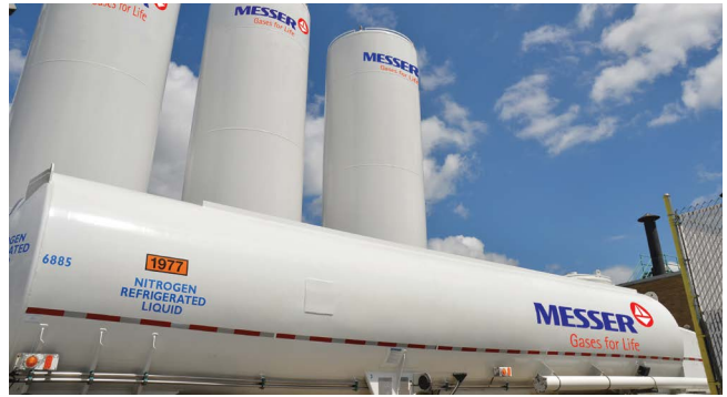
Liquid nitrogen is supplied by truck to storage silos, owned and maintained by Messer, outside Nation's nearly 200,000 sq. ft. production facility in Schaumburg, IL.
