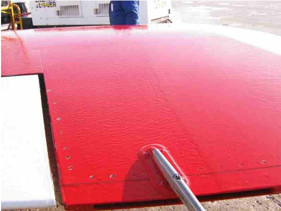
Photo 4.1: Residual Fluid on Trailing Edge
