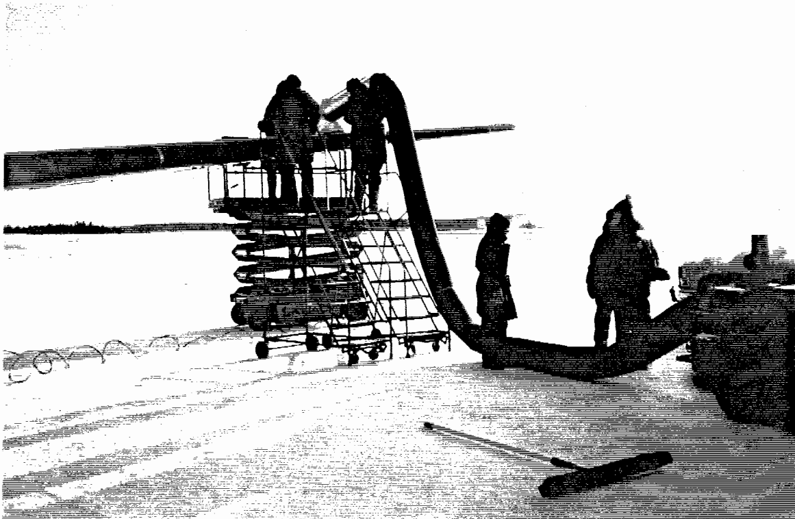
PHOTO 2 HOT AIR APPLICATION EQUIPMENT
