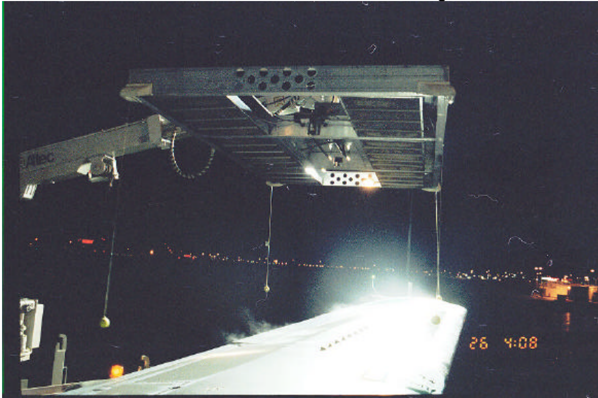
Photo 2.3 Heater Panel Positioned over the Wing
