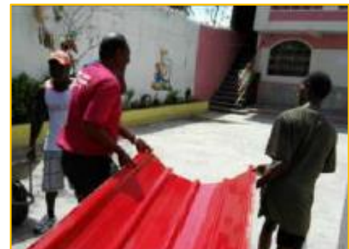
A classroom that lost its roof (top), HOPEww distributing roofing in Les Cayes (bottom)
