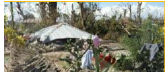
Pictured above: Houses destroyed or damaged in the South Department of Haiti
