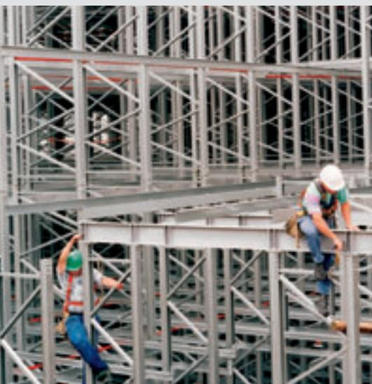
Warehouse systems are designed for use in warehouses or as “Rack supported structures”. For the silo construction, the racking is mounted on a concrete base in the open air. The racking is then clad with walls and roof.
