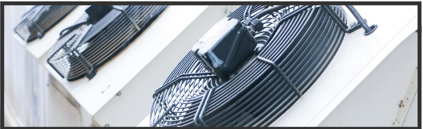
The performance of air conditioning equipment improves in direct proportion to how well the unit matches the application. There is a common but erroneous belief that oversizing the unit is preferable, so that it can cool indoor spaces faster while reducing the compressor runtime. However, this comes with many performance issues. Also, even though the compressor runs less time, it also draws more power than a properly sized unit, so energy savings are minimal or zero.
