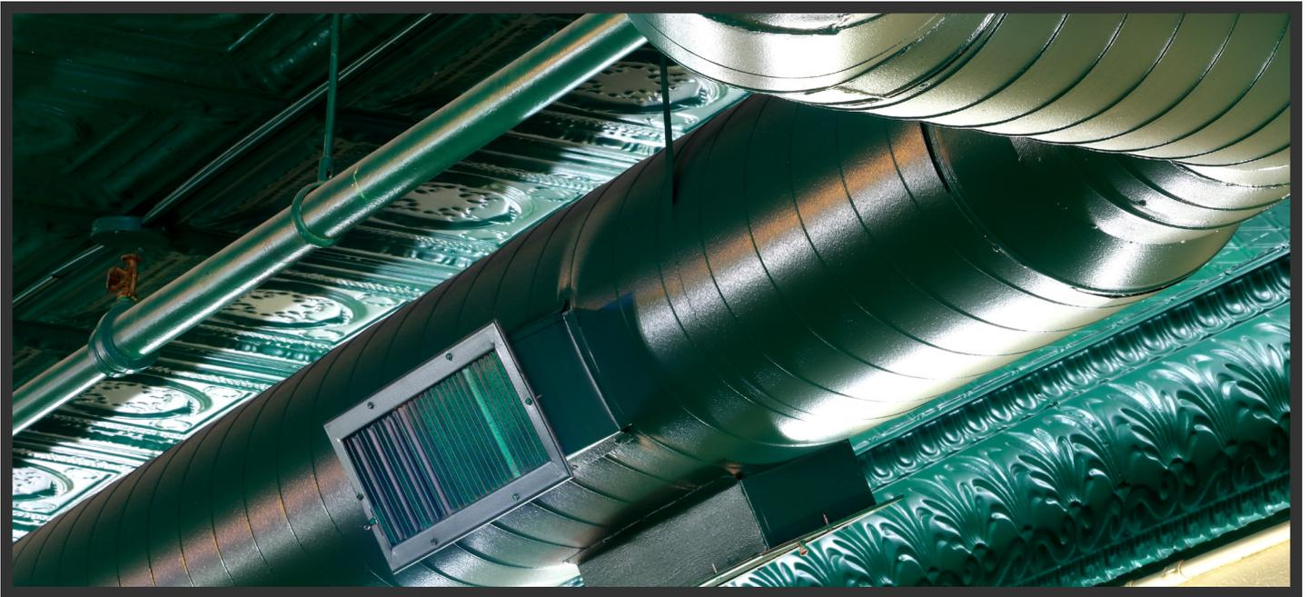
Both pressure drop and velocity decrease as the cross-sectional area of a duct becomes larger, but there is an upper limit to how much duct size can be increased.
