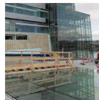
CURTAIN WALL INSTALLATION REVIEW
