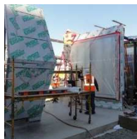
CURTAIN WALL MOCK-UP REVIEW
