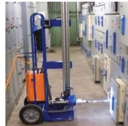
**Roll-up Racking with Full Breaker Removal Tools:** Variations on roll-up style may be equipped with an extraction type mechanism for breaker insertion and removal in conjunction with jack accessories to lift and transport a large circuit breaker. For large medium voltage and heavy air frame circuit breakers, varieties can also incorporate a crane for hoisting and support for these heavier circuit breakers.
