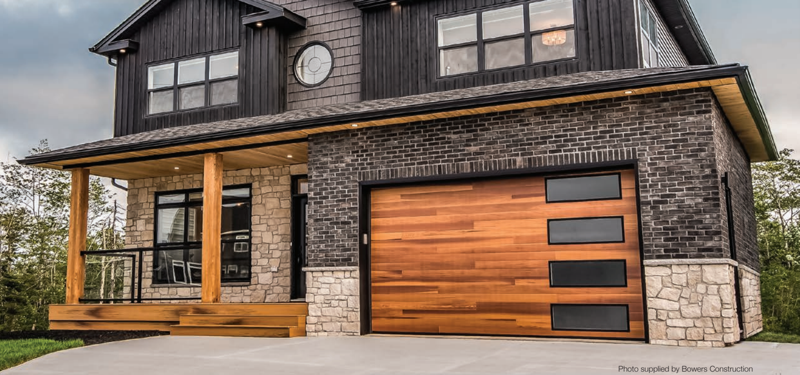
Photo supplied by Bowers Construction
