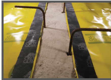
At Interior Grade Beam Impediments: Install Stego Crete Claw onto the terminating edge of Stego Wrap.
