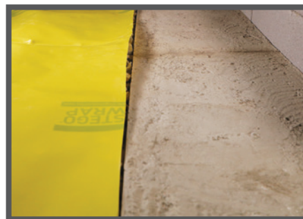
Note: The distance to which the vapor barrier is extended adjacent to, onto, or completely over a footing or grade beam should be determined by the project design team.
