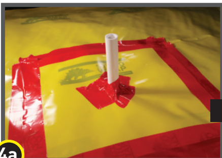
1 Cut a detail patch to a size and shape that creates a 6" overlap on all edges around the void space at the base of the pipe.
