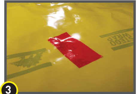
3 Center Stego Tape over small hole or slice in Stego Wrap.
