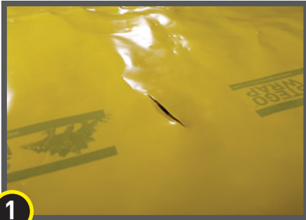
1 Small hole or slice in Stego Wrap.
