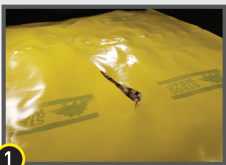
Occasionally there are larger holes in the vapor barrier that require a patch.
