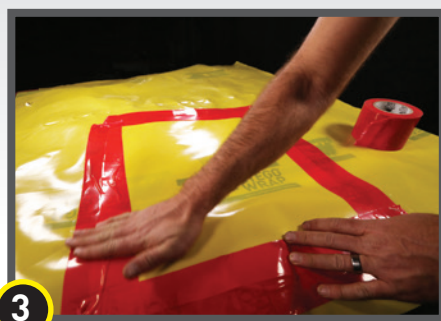
Measure and cut a piece of Stego Wrap to cover damaged area 6" in all directions. Seal patch with Stego Tape.
