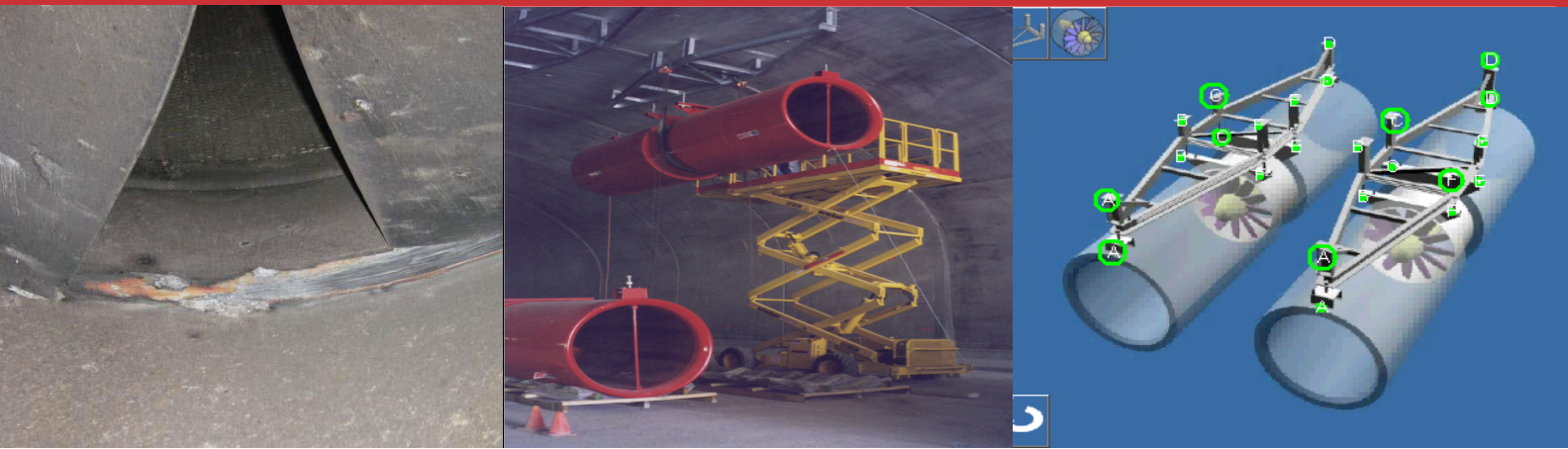
Pictured: 1. An example of fan blade wear and tear. 2. Installation in progress. 3. Screen monitor shows sensors (green) on the fans.
