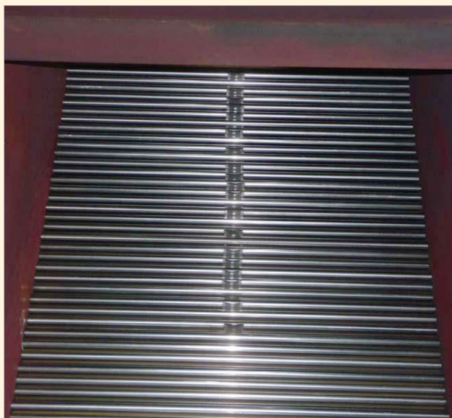
Figure 13. Partially staked bay
