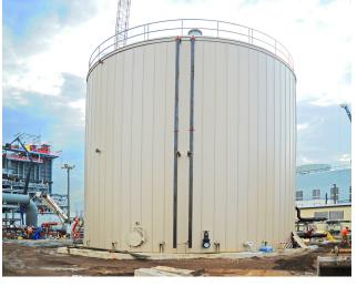
Fisher Tank Company provides engineering, fabrication and construction for field erected welded steel Thermal Energy Storage tanks.
