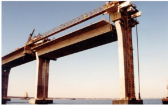
1986: Jamestown Verrazano Bridge, RI VSL
