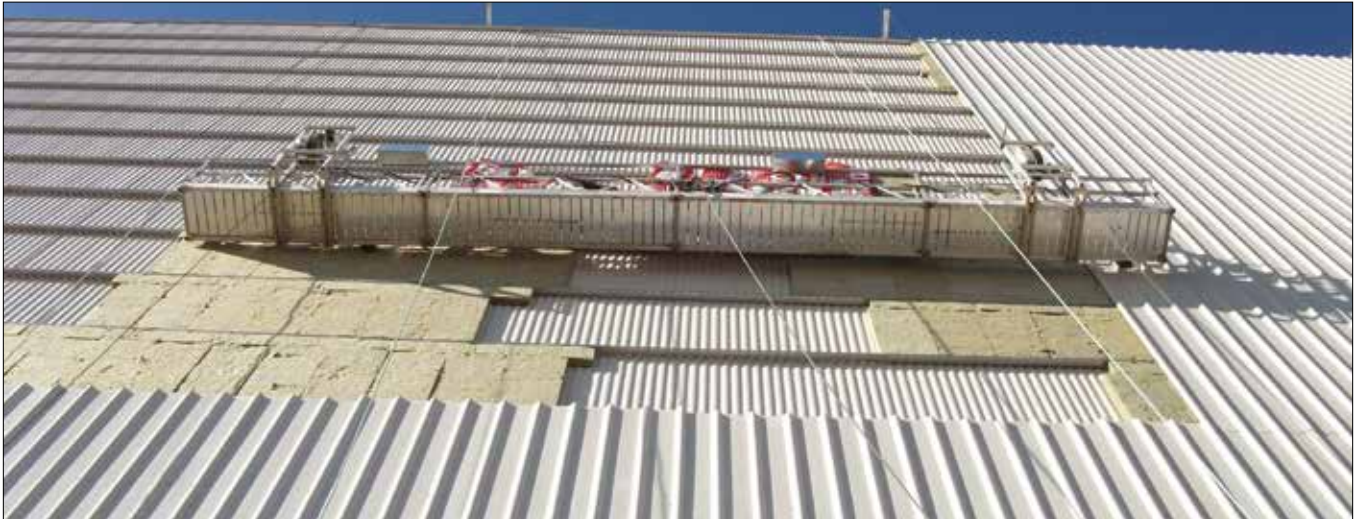
Tuff Span insulated panel system at potash operation. Assembly includes liner, stainless steel sub-girt, mineral wool insulation, and exterior sheet.
