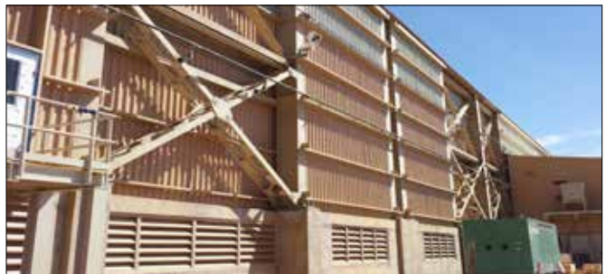
Tuff Span Louvers, Beams & Cladding at copper mine
