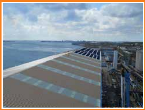
Tuff Span opaque and translucent cladding, beams, louvers, and gutter at Desalination plant
