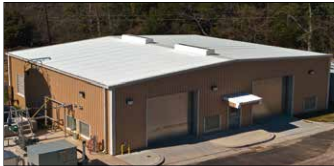
Tuff Span 12" Ridge Vent installed with FRP cladding, louvers, gutter.
