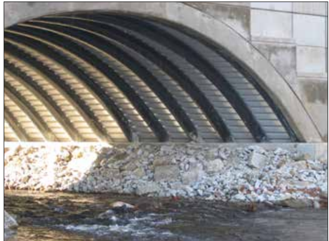
Tuff Span Form Deck for road bridge
