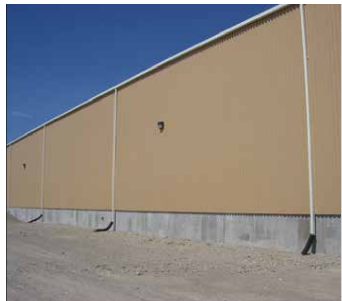
Tuff Span gutter, downspout, roofing, and siding at metal alloy processing plant
