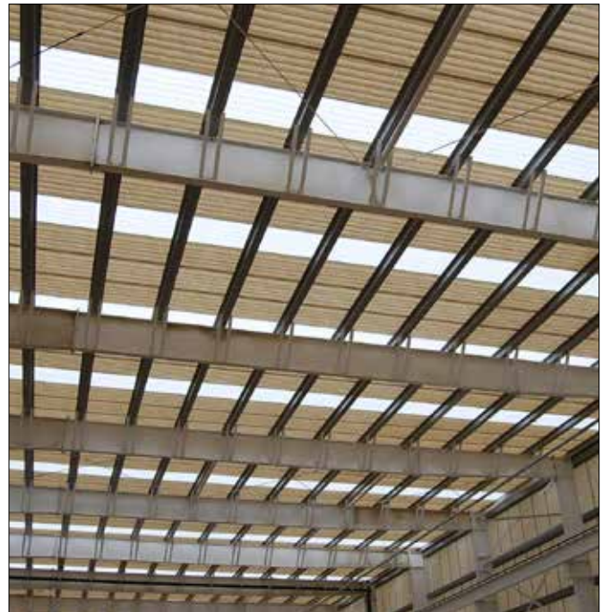
Tuff Span Roofing, Siding, and Purlins at metal treatment plant
