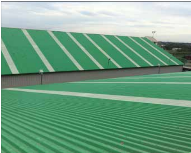
Tuff Span opaque & translucent cladding at fertilizer blending facility.
