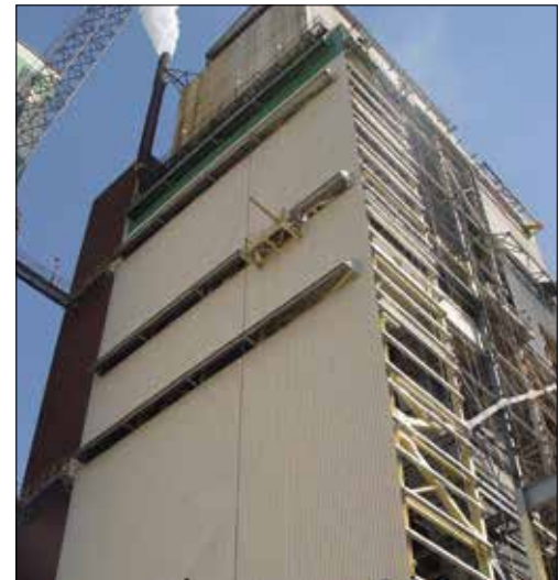
Tuff Span FM siding on 130 foot tall recovery boiler at coastal location
