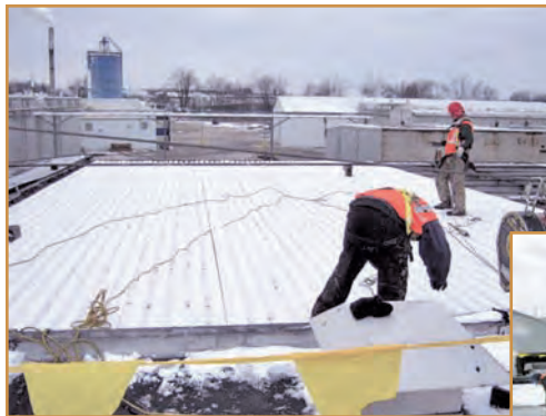
Photo 2 – Fastening of FRP roof deck to supports is similar to a metal deck. Layout of the lighter FRP sheets is faster.
