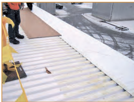
Photo 5 – FRP roof decks are a suitable substrate for either single-ply or built-up roofing.
