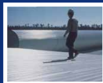
Tuff Span panels at aluminum smelter
