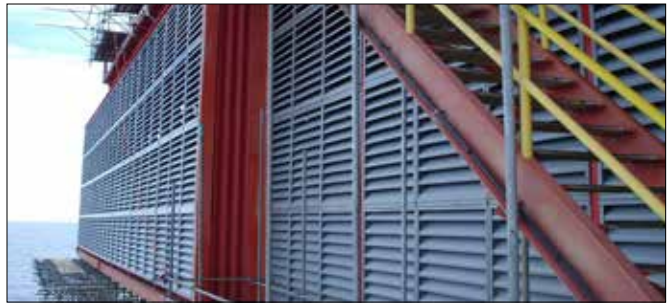
Tuff Span Louvers & Windwall Panels at offshore platform
