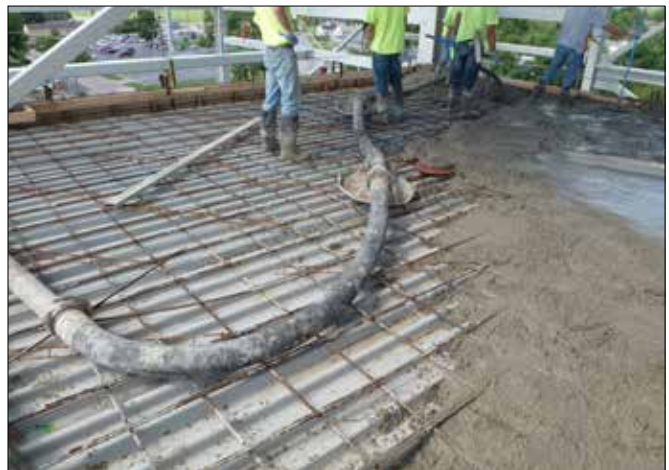
Tuff Span Form Deck at food processing plant
