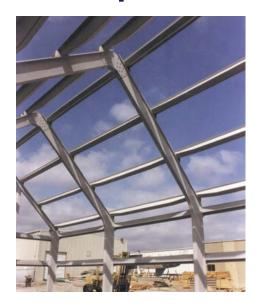
Enduro offers standard and custom shapes for challenging, structural and environmental conditions. Delivering long, maintenance-free service life, the structural sections are cost effective solutions for industrial buildings in corrosive environments.
