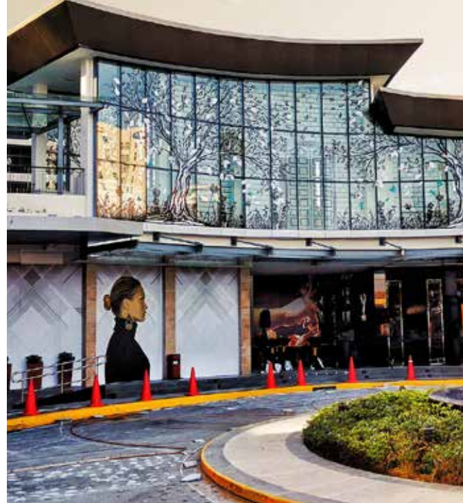
Image: Courtesy of H.S. Pow Construction and Development Corporation
