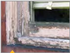
This window and its original wooden frame are in poor condition, showing signs of rot. In a typical pocket replacement, the rotted trim and frame may be covered with aluminum coil, leaving a dark, moist environment where mold can thrive.
