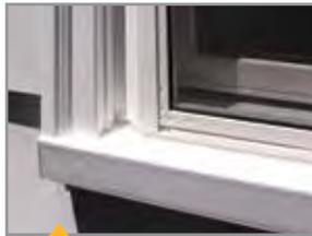
With Full Frame Replacement, the old, deteriorated brickmould and framing is removed, and a new decorative brickmould would be installed, providing a structurally sound, rejuvenated, moisture-free frame for the new window.
